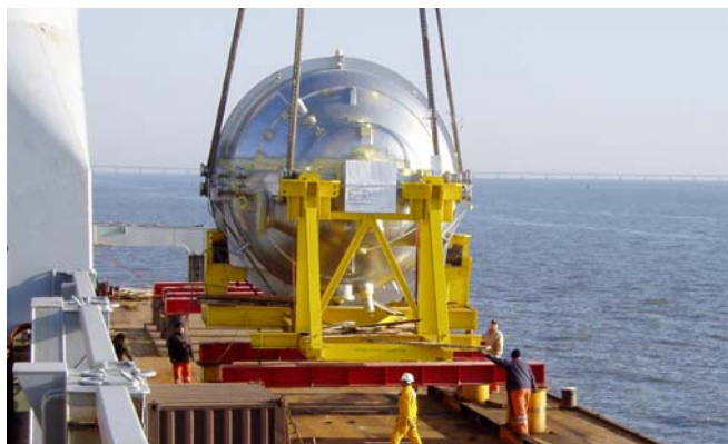
Steam turbine shipment from overseas
